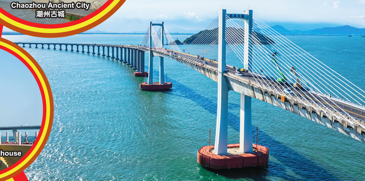
Nan'ao Bridge 南澳大桥
